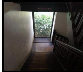
Wood from rafters reused for window frames
