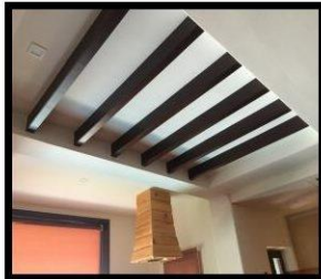
Wood from rafters reused to decorate ceiling
