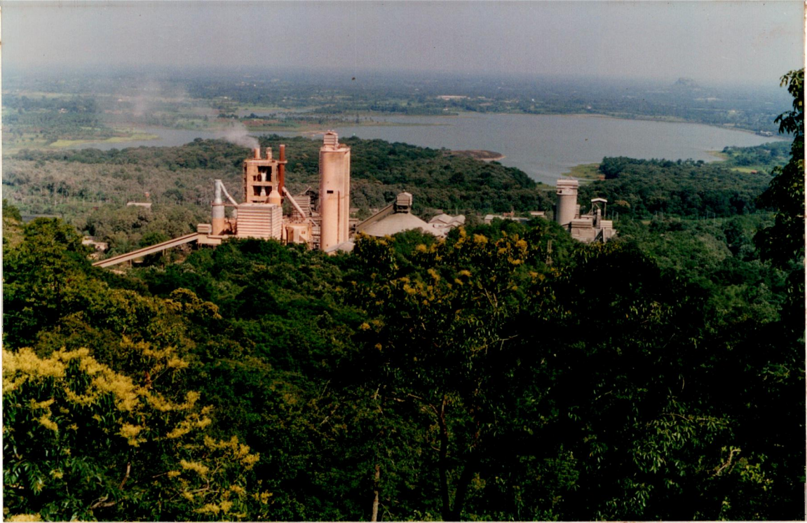
FIGURE 2 AERIAL VIEW OF MALABAR CEMENTS LIMITED, WELAYAR
