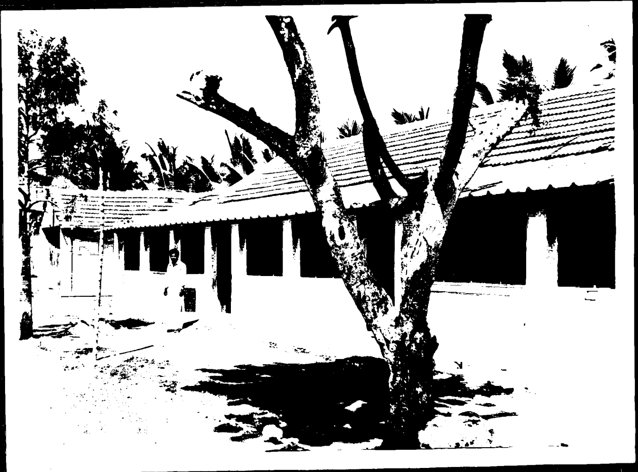
FIGURE-4a. BEFORE PUTTING UP OF THE COMPOUND FENCING AND GATE [SCHOOL]
