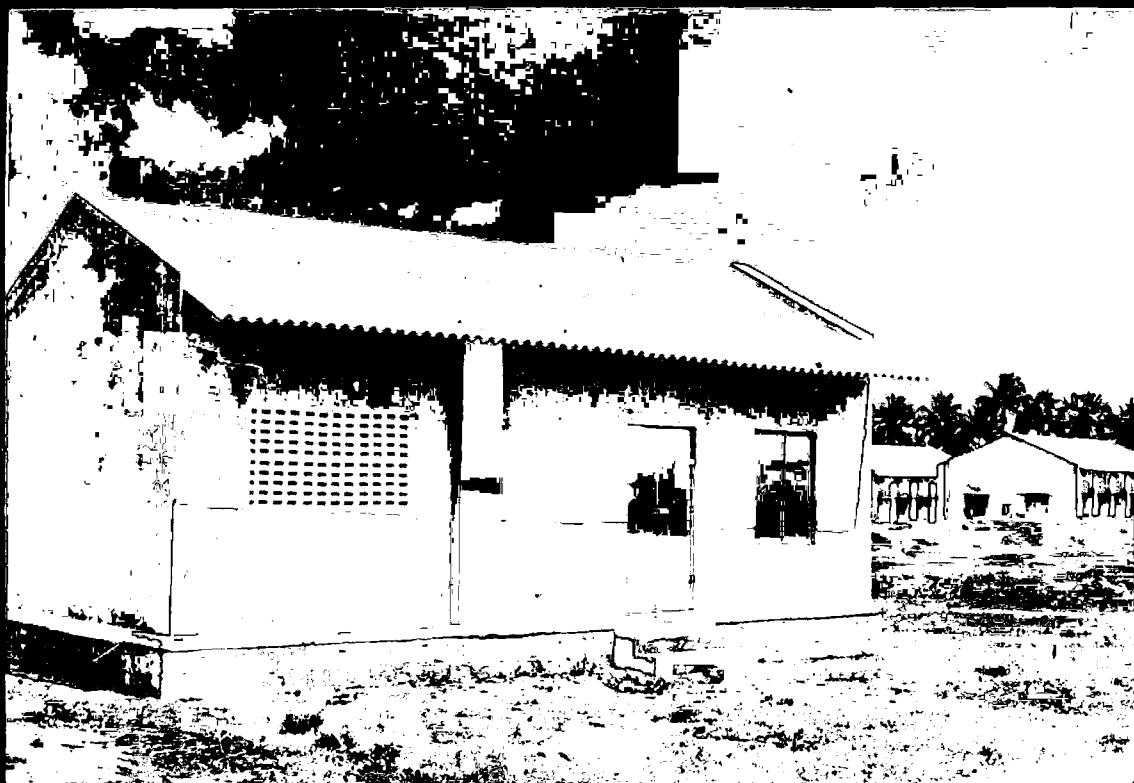
FIGUR IV COMMUNITY HALL UNDER NREP
