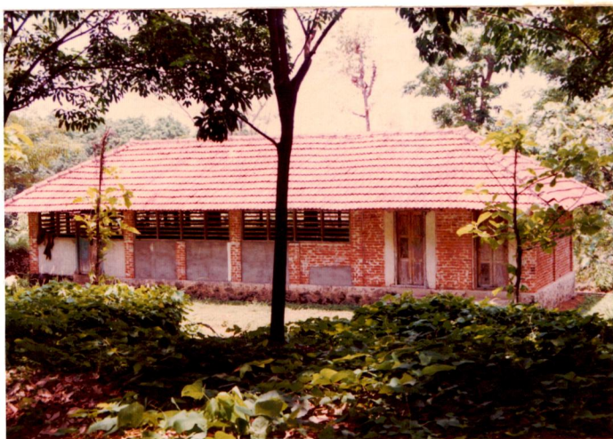
Latex processing unit
