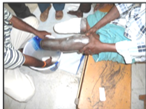
Plate -1 Socket fabrication process
