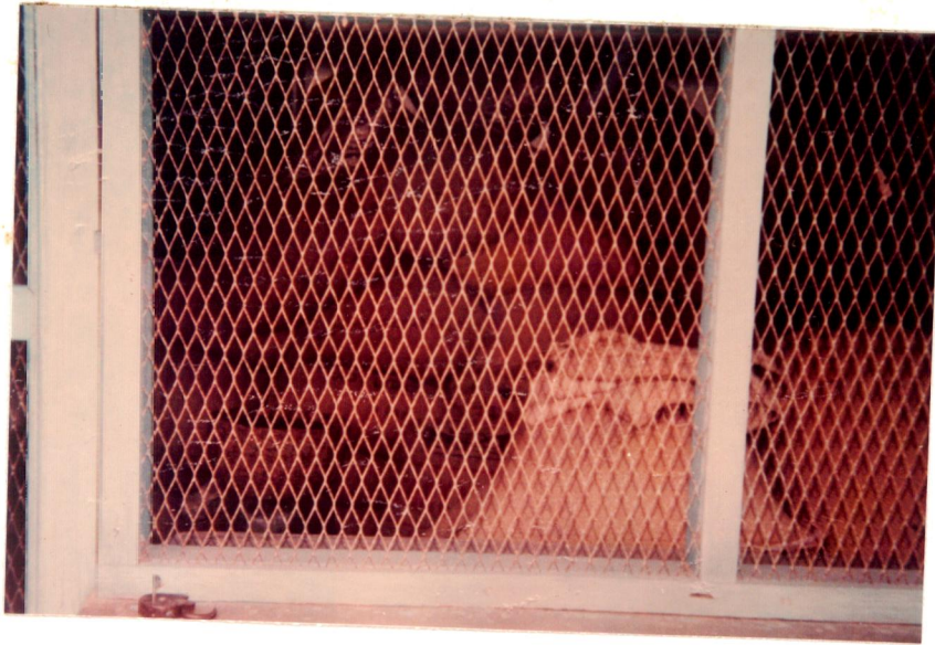
Plate - 9 Wire Mesh Fitted Window
