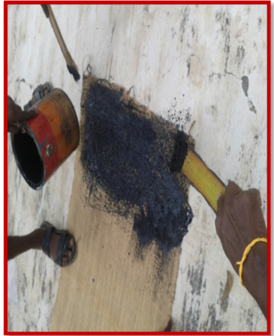
Plate IX: Application of Bitumen
