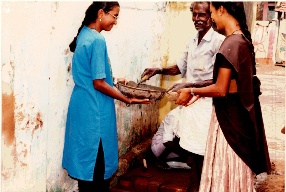
FIG 4 CONSTRUCTION OF TOILET FOR ANGANWADI
