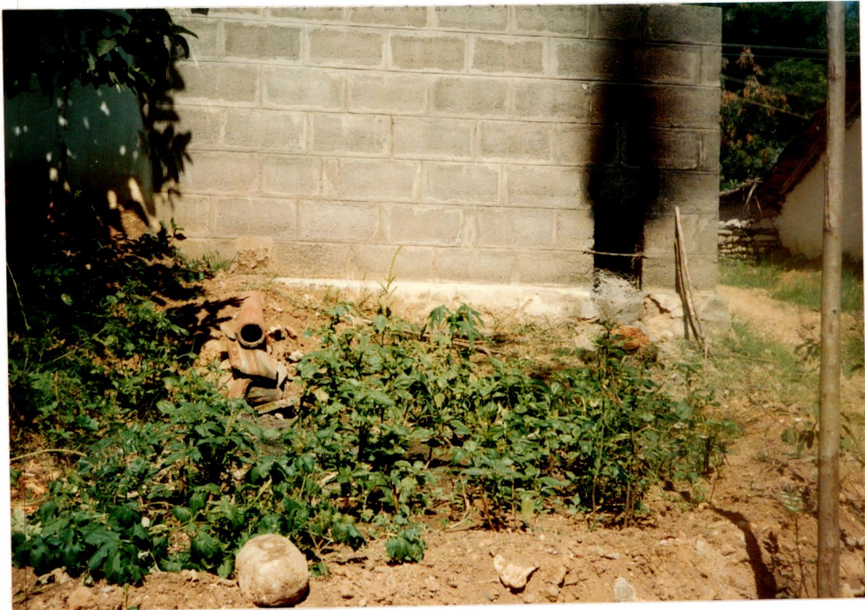
KITCHEN WASTE WATER DIVERTED FROM KITCHEN OUTLET FOR RAISING KITCHEN GARDEN
