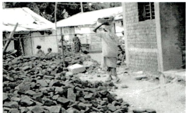
Figure 2: Worker's showing the Distance Traversed
