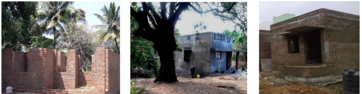
Plate 16 : Green House Construction in Progress (CMSPGHS).
