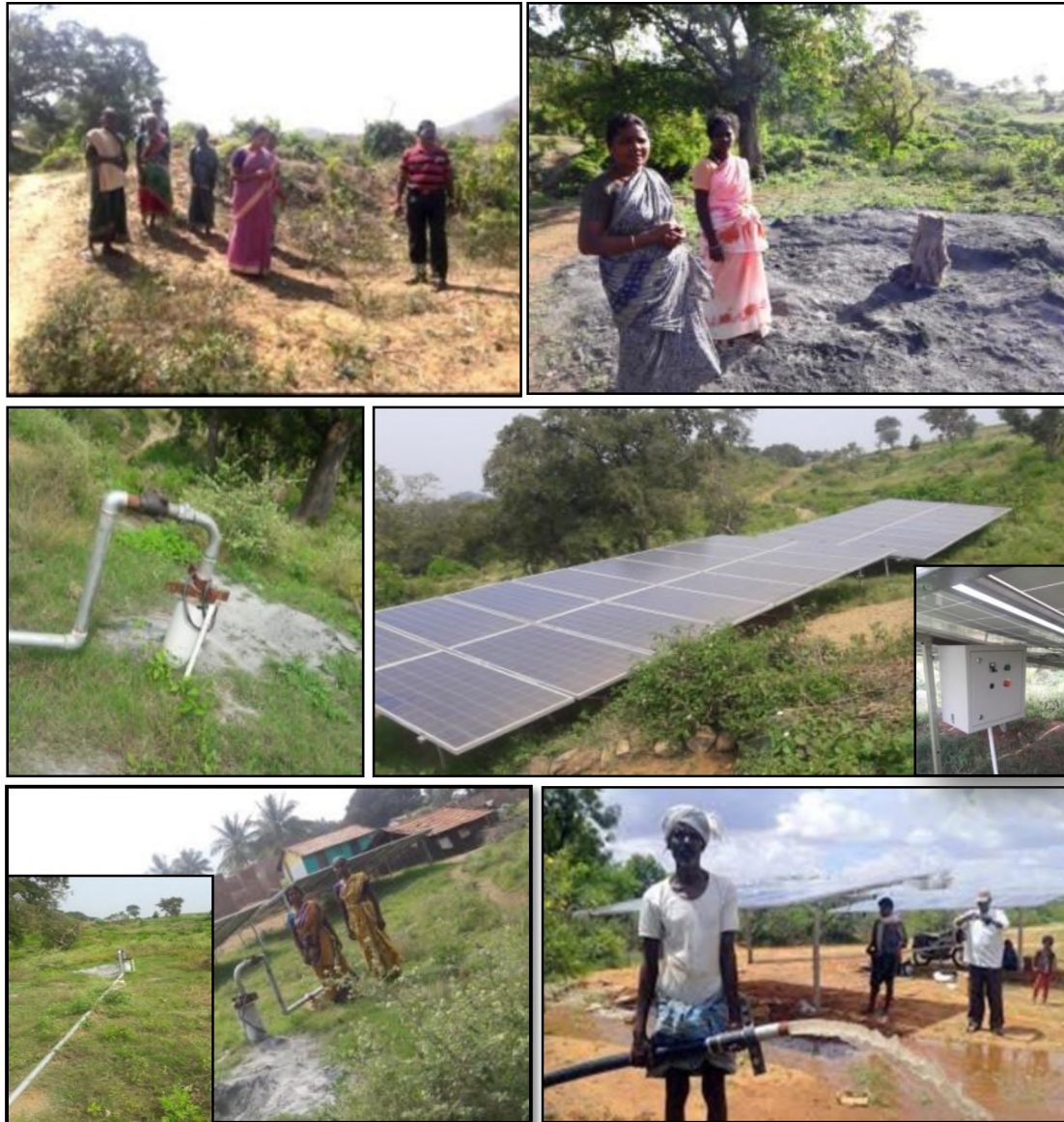
Plate: 17 Installation of Solar Bore well Plant under THAI Scheme (Tamil Nadu village Habitations Improvement Scheme)
