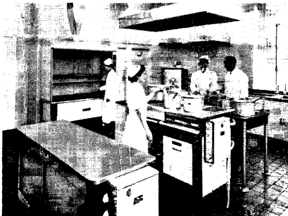
15. Electrical cooking for Executives' dining room, Central Electricity Authority Headquarters, London
