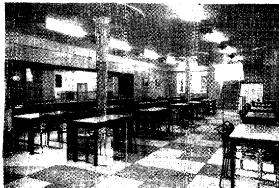
12. Terrazzo flooring in the Baker Street canteen of London Transport Executive
