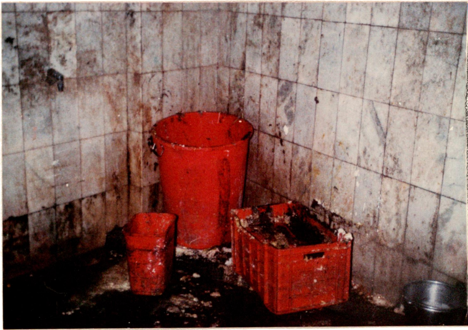
PLATE V - WASTE DISPOSAL UNIT IN HOTEL B
