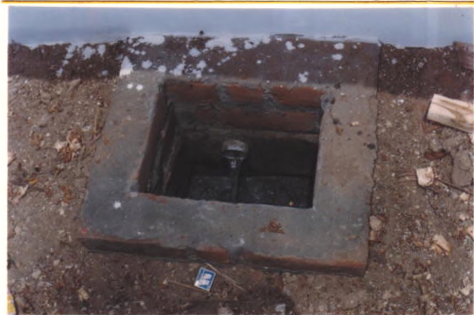
Constructed Soakpit
