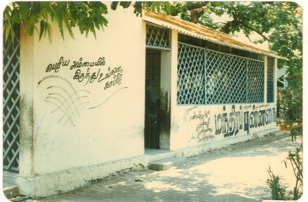
Picture 6 An Anganwadi Building
