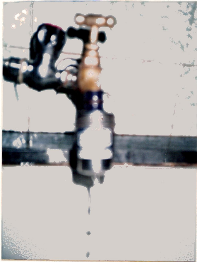
PLATE 11 - POLYIODIDE RESIN PORTABLE FILTER ATTACHED TO THE TAP
