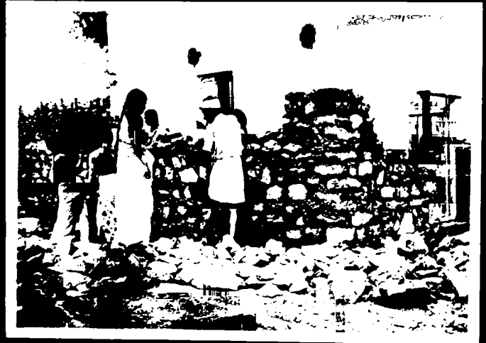
CONSTRUCTING SCHOOL LUNCH KITCHEN
