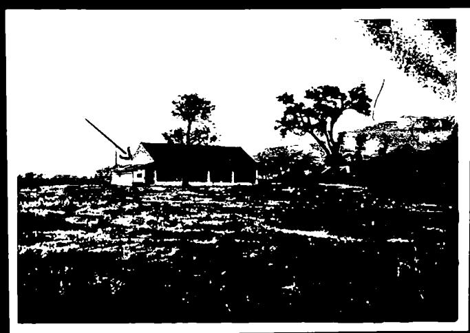
A VIEW OF THE KITCHEN CONSTRUCTED
