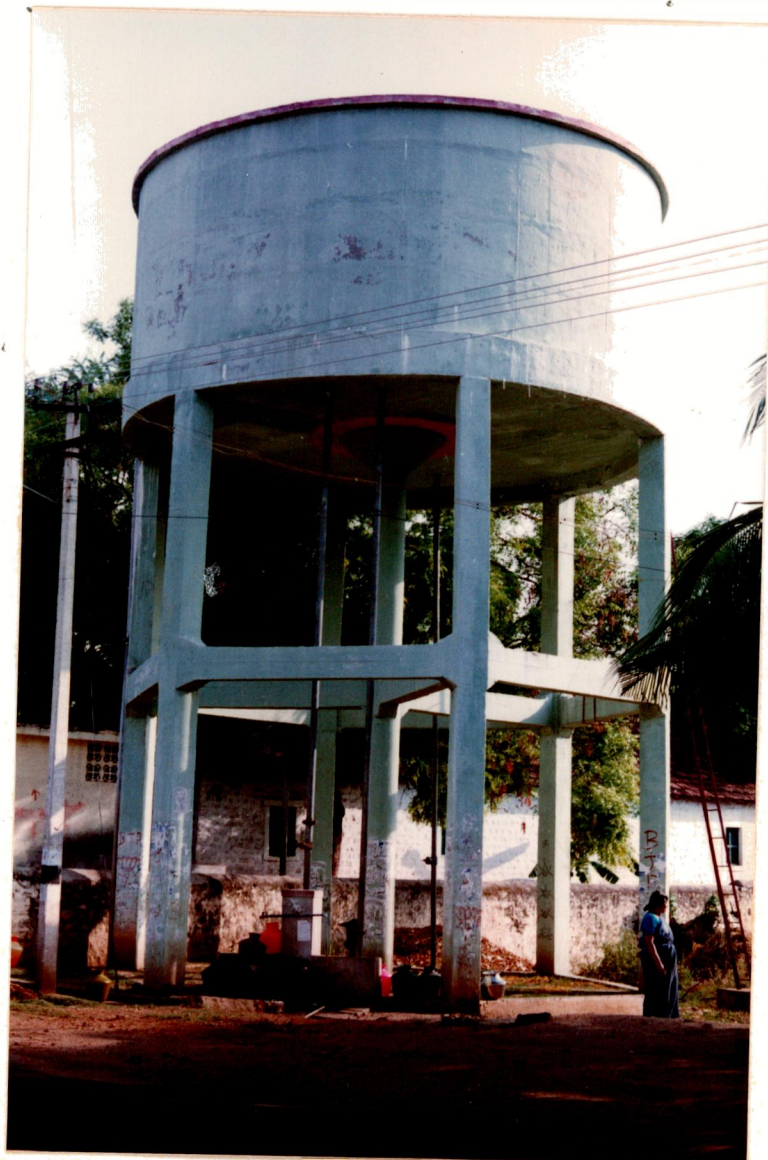
Fig.III The bore well at Lakkapuram Village.
