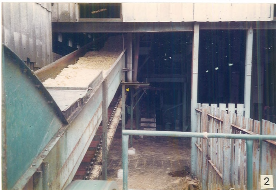
Crushed cane passed to water boiler
